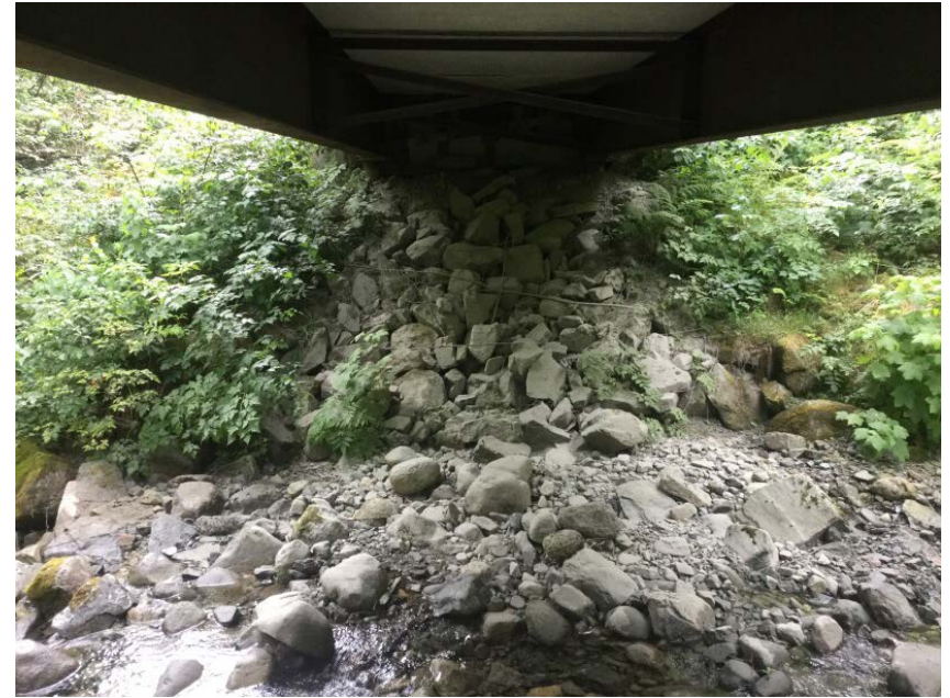
Right Bank Abutment when facing downstream
