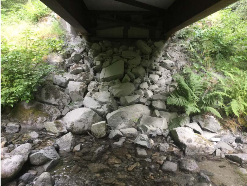
Left Bank Abutment when facing downstream
