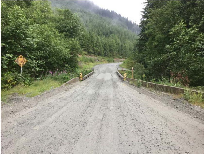
Approach from Right Bank when facing downstream
